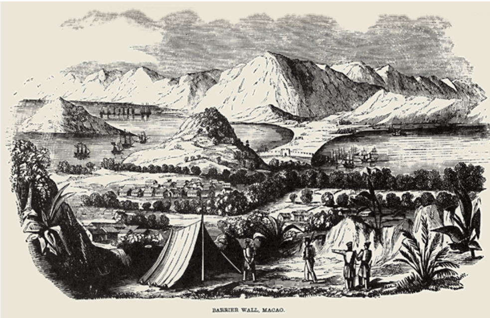
BARRIER WALL, MACAO.
