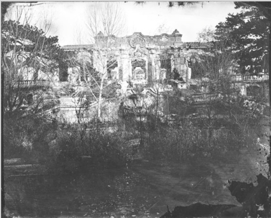
Haiyantang, west façade
