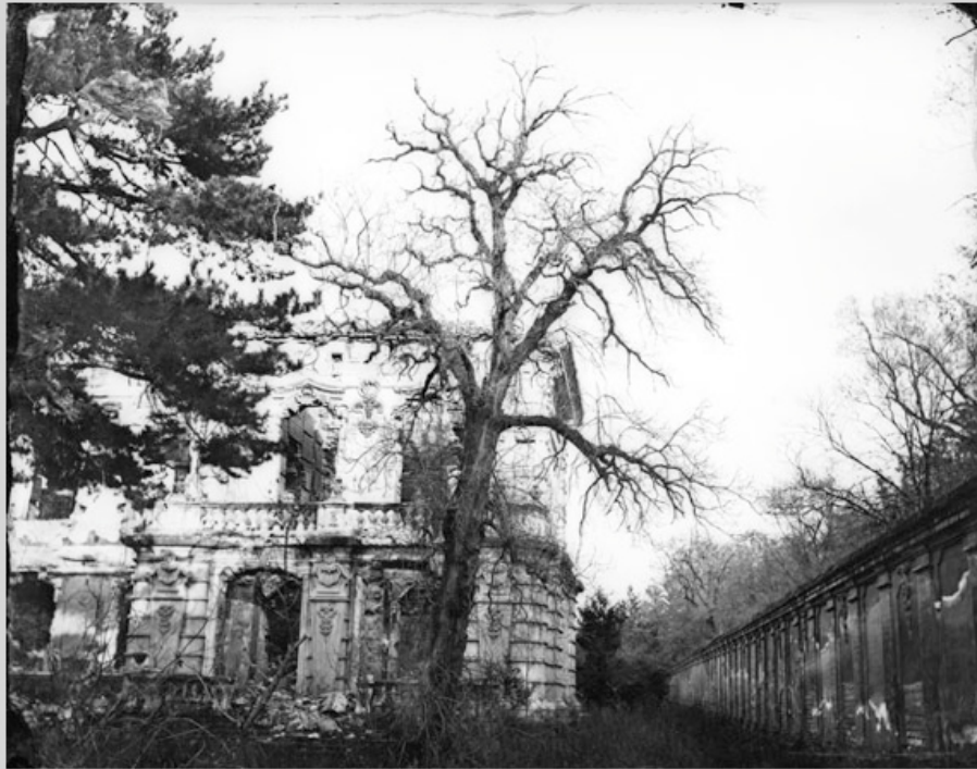
Haiyantang, north façade
