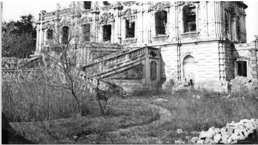
Xieqiqu, south façade Built in 1751, this was the first pavilion in the Xiyanglou. Depicted in Engraving 1.
