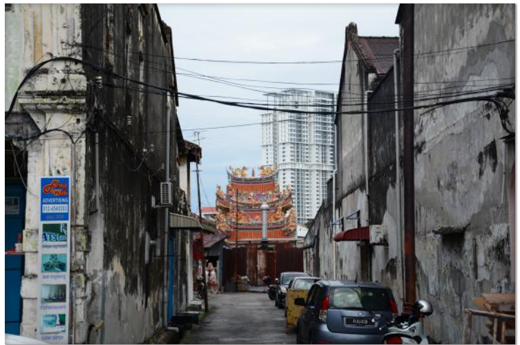
Figure 27. A typical street with dilapidated shop houses in George Town, with new, high-rise housing development in the background. Photo Credit: Sera Tolgay, 2017
